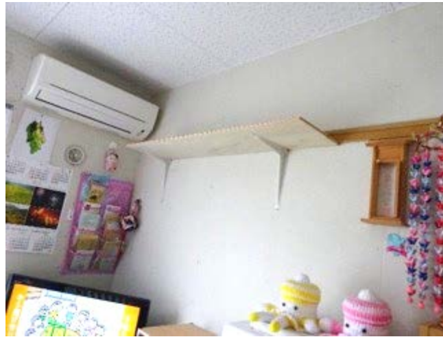
Shelf installation at a temporary housing
